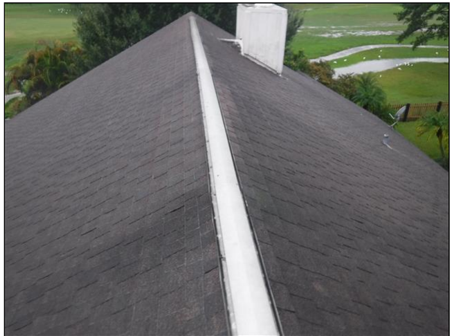
View of Roof While Walked
