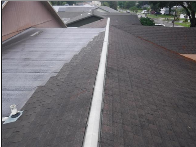
View of Roof While Walked
