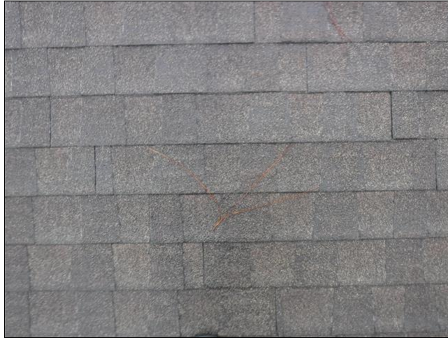
View of Roof While Walked
