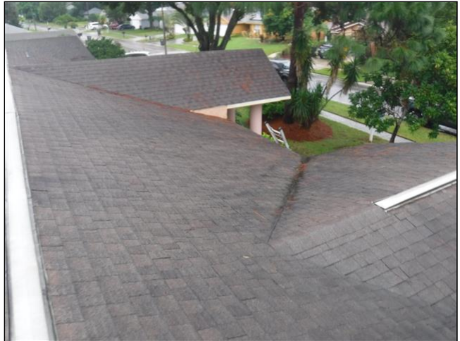
View of Roof While Walked
