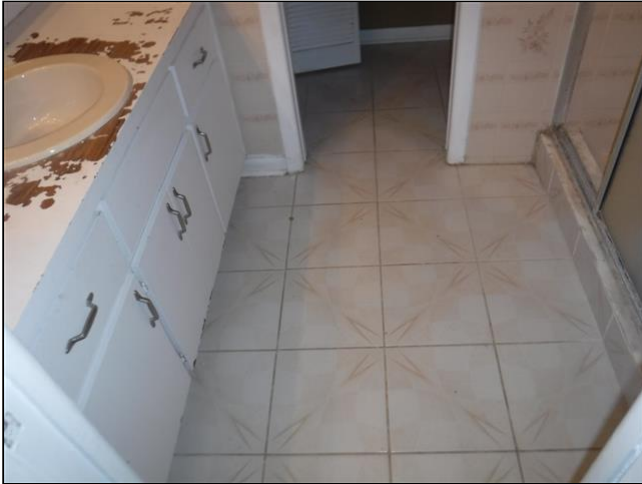
Old Master Bathroom
