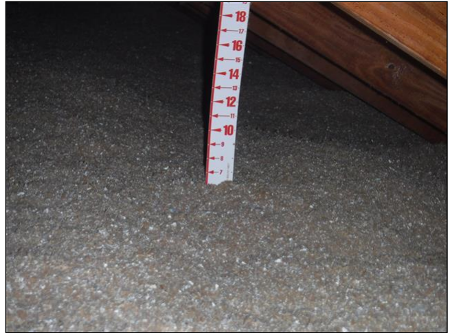
Photos of Attic Space
