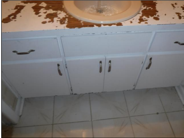
Old Master Bathroom
