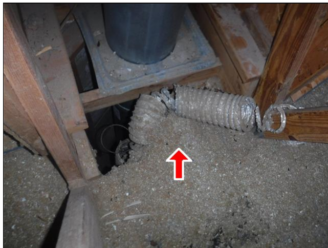
Photos of Attic Space
