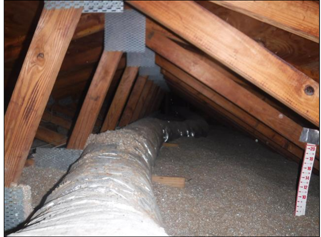
Photos of Attic Space
