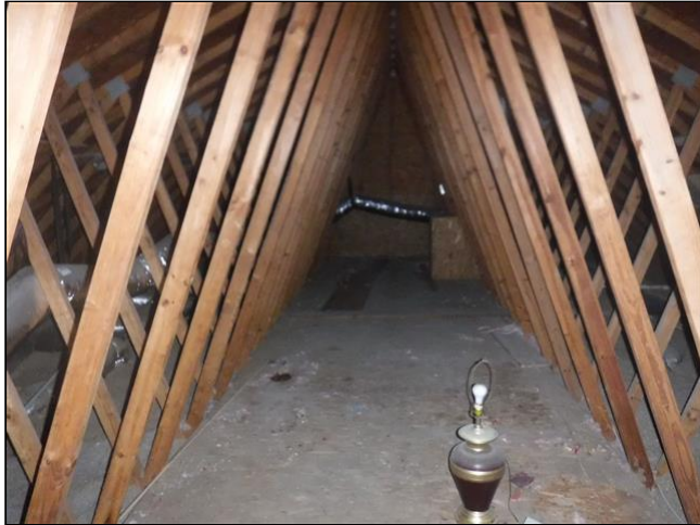
Photos of Attic Space
