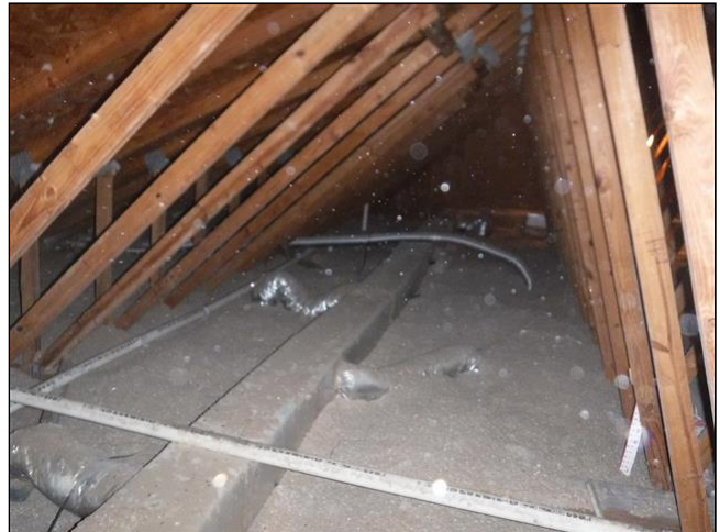
Photos of Attic Space
