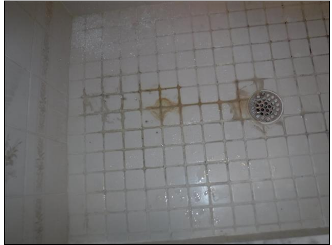
Old Master Bathroom
