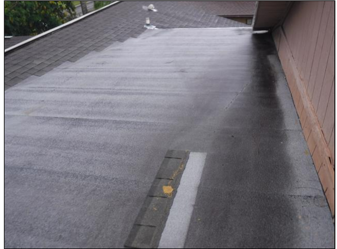
View of Roof While Walked
