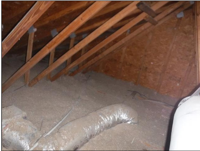
Photos of Attic Space
