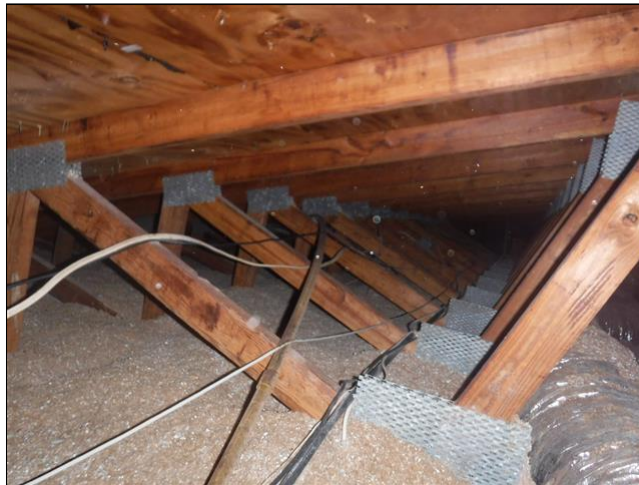
Photos of Attic Space
