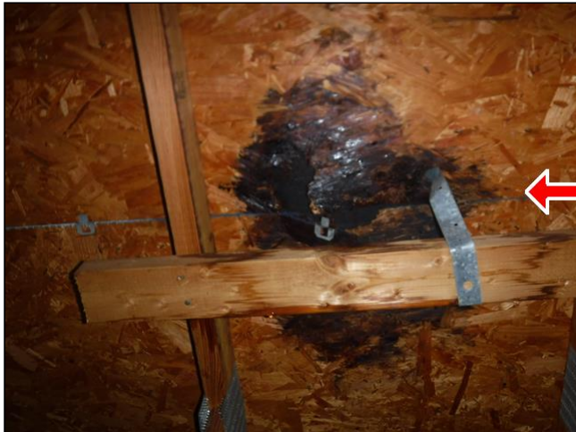
Photos of Attic Space
