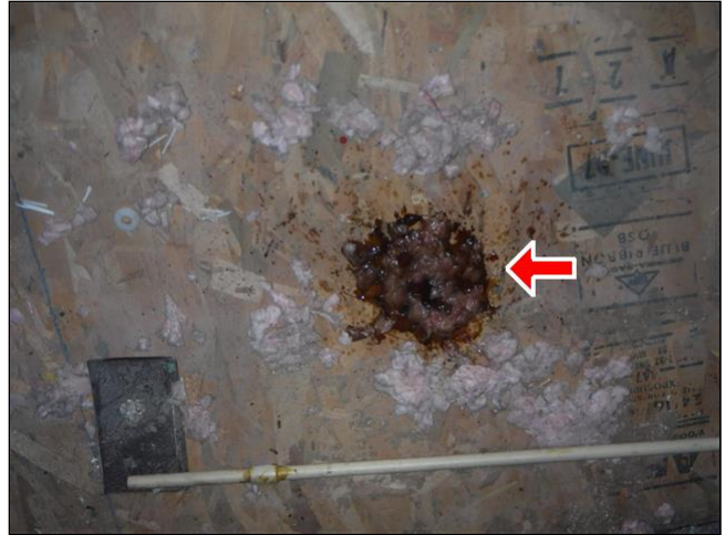
Photos of Attic Space
