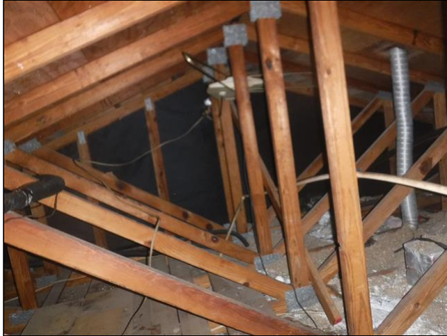
Photos of Attic Space
