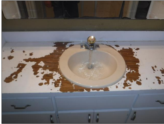
Old Master Bathroom
