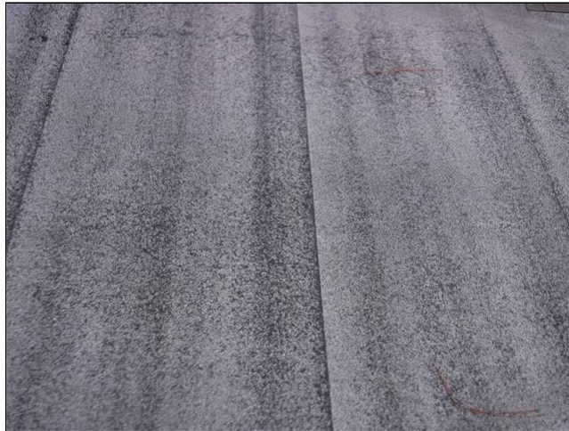
View of Roof While Walked
