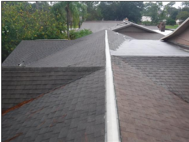
View of Roof While Walked
