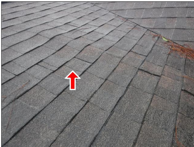
View of Roof While Walked
