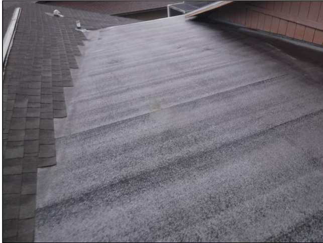
View of Roof While Walked
