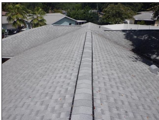
View of Roof While Walked
