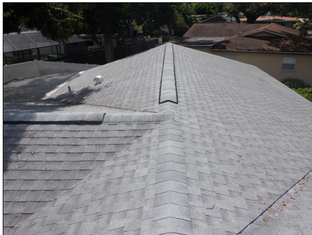
View of Roof While Walked
