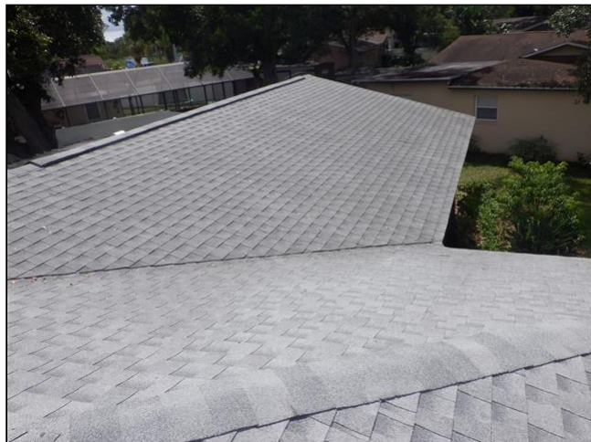
View of Roof While Walked
