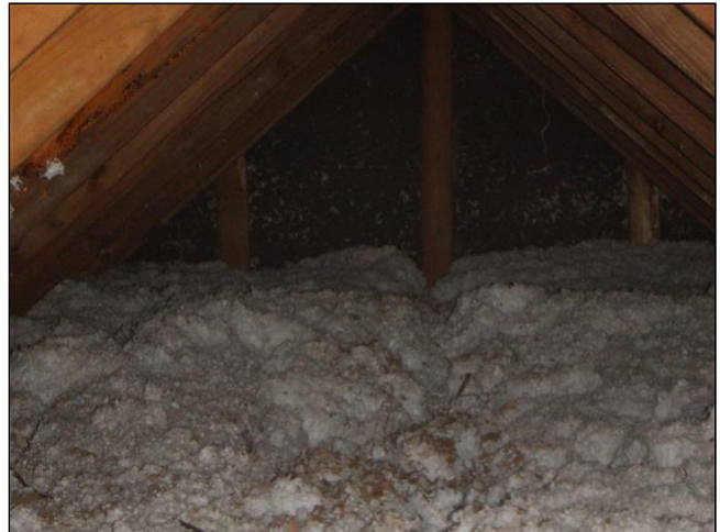
Photos of Attic Space
