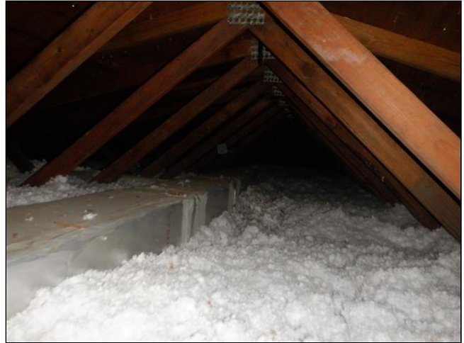
Photos of Attic Space
