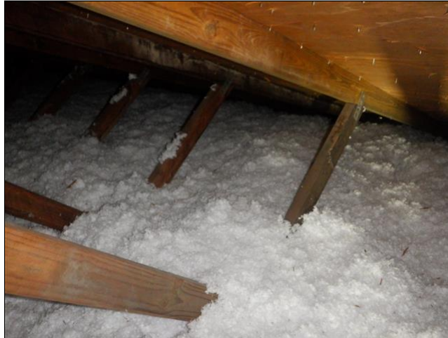
Photos of Attic Space
