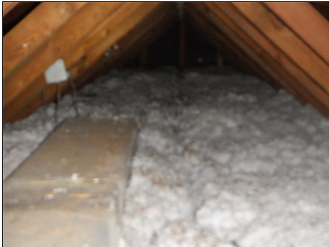
Photos of Attic Space
