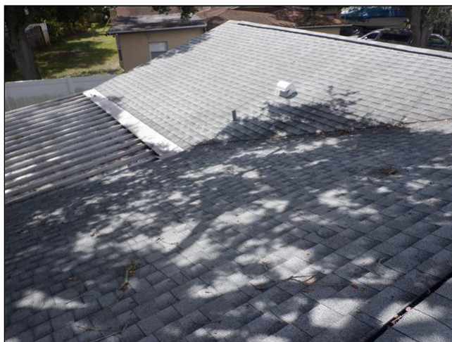
View of Roof While Walked
