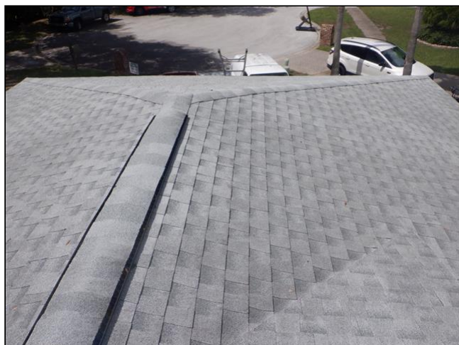
View of Roof While Walked
