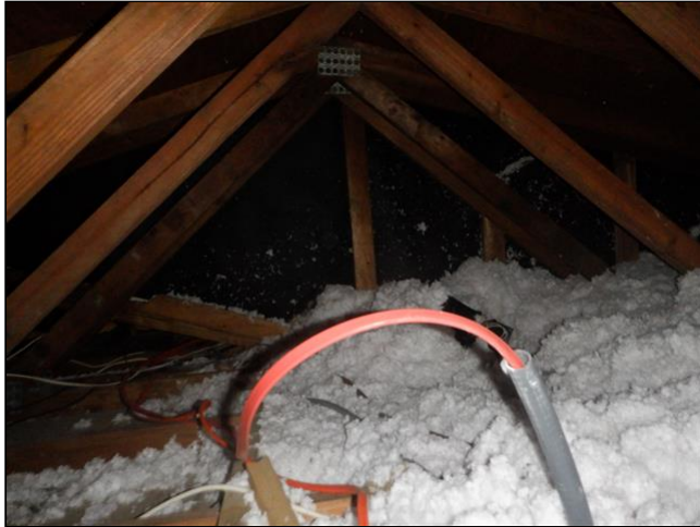
Photos of Attic Space
