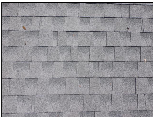
View of Roof While Walked
